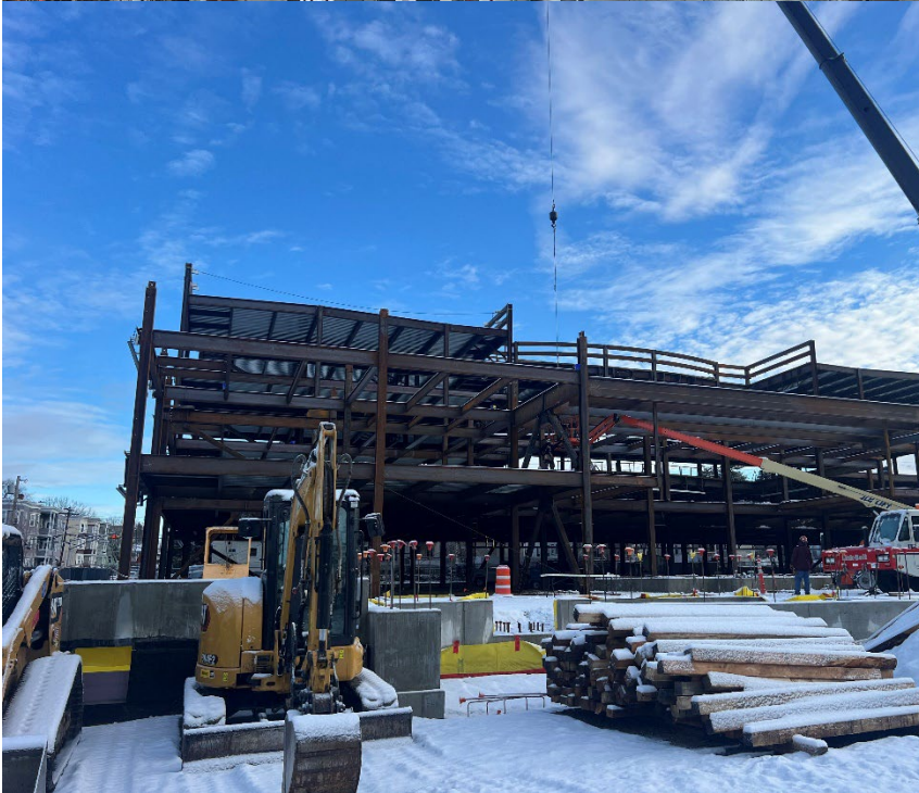
Progress photo at the end of the month (1/29/24).
