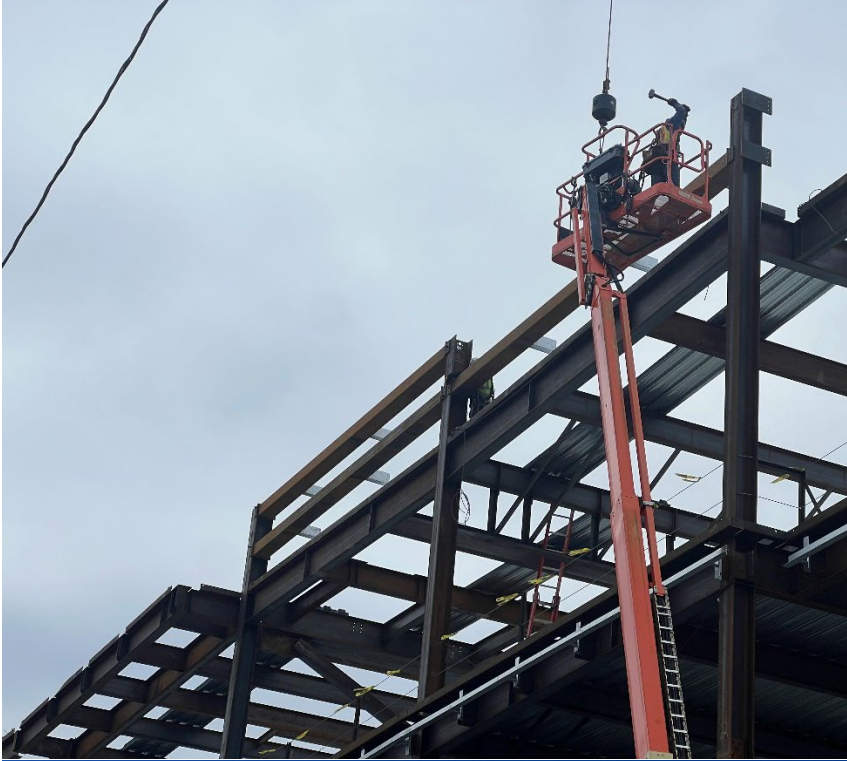
Installation of steel for the parapet.
