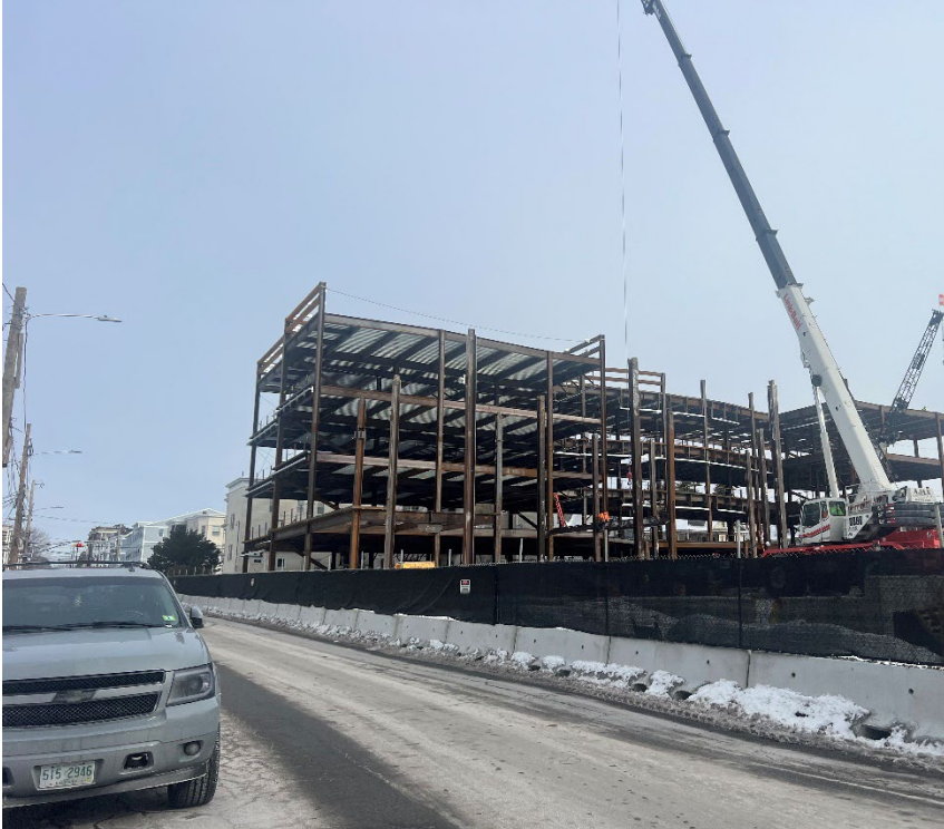
Beginning of Phase 2 of the steel erection.
