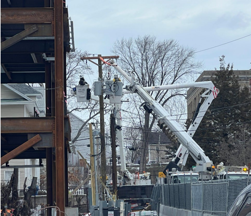
National Grid on site installing transformers on the new pole.
