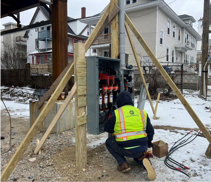
Electrician from Griffin Electric installing the temporary power panel.
