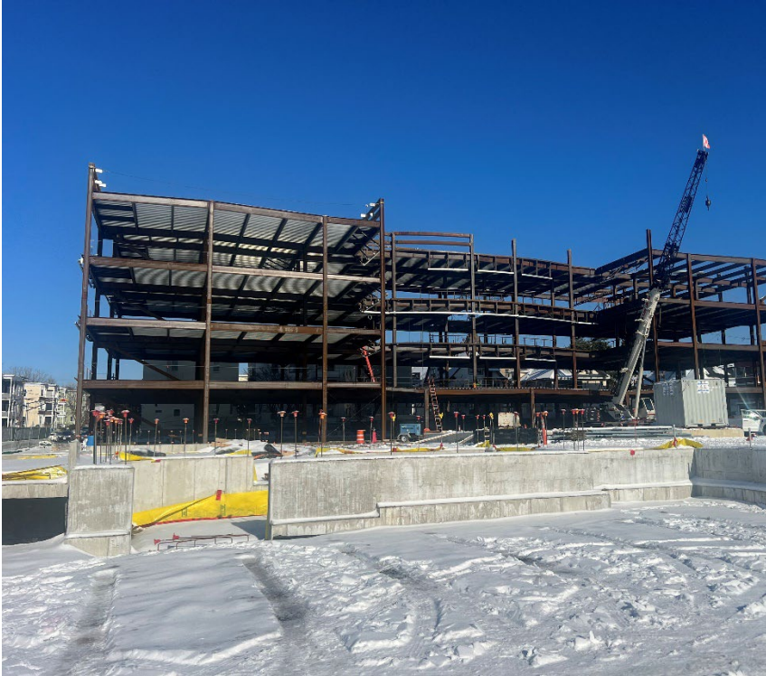
Overall photo of progress mid-month (1/17/24).
