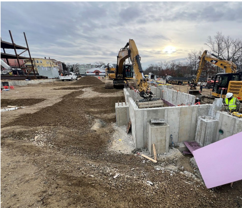
Backfilling of the building interior.
