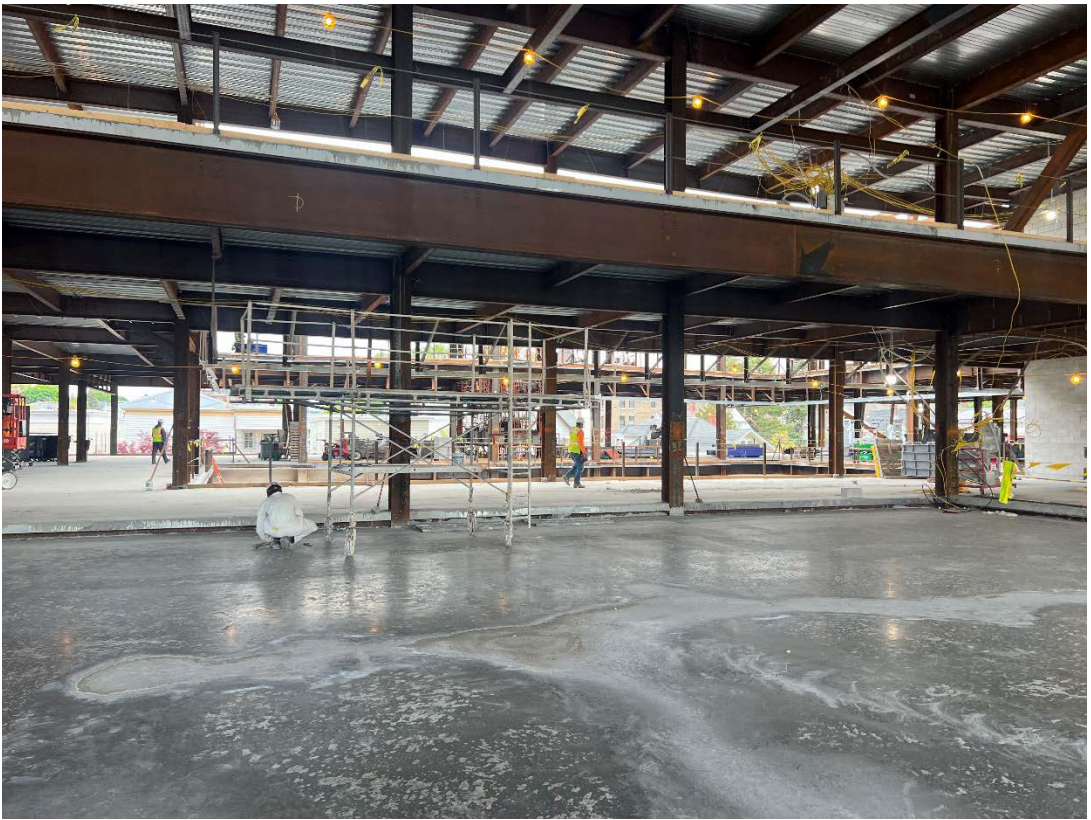
3 rd floor looking through the building from across the gym.
