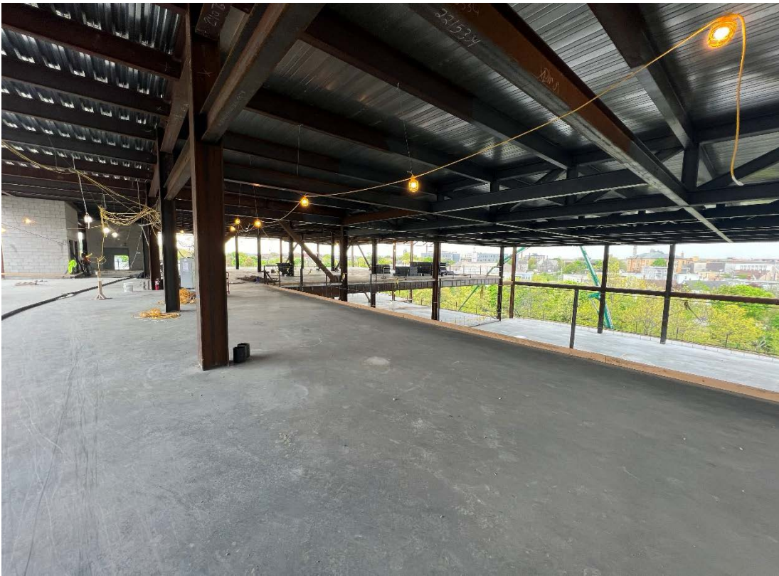
4 th floor view.
