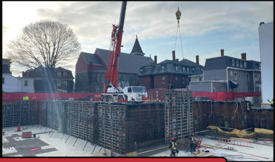
Gang Form Install for Foundation Walls
