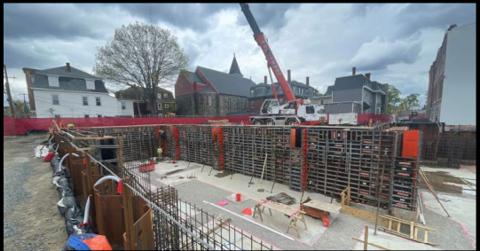
Gang Form Install for Foundation Walls
