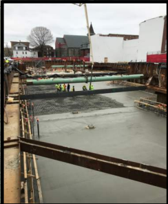
Concrete Mat Slab Placement #3 (West)
