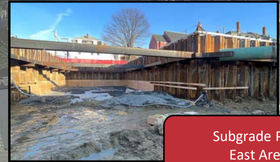
Soil Excavation for 2 nd Cut Center Area
