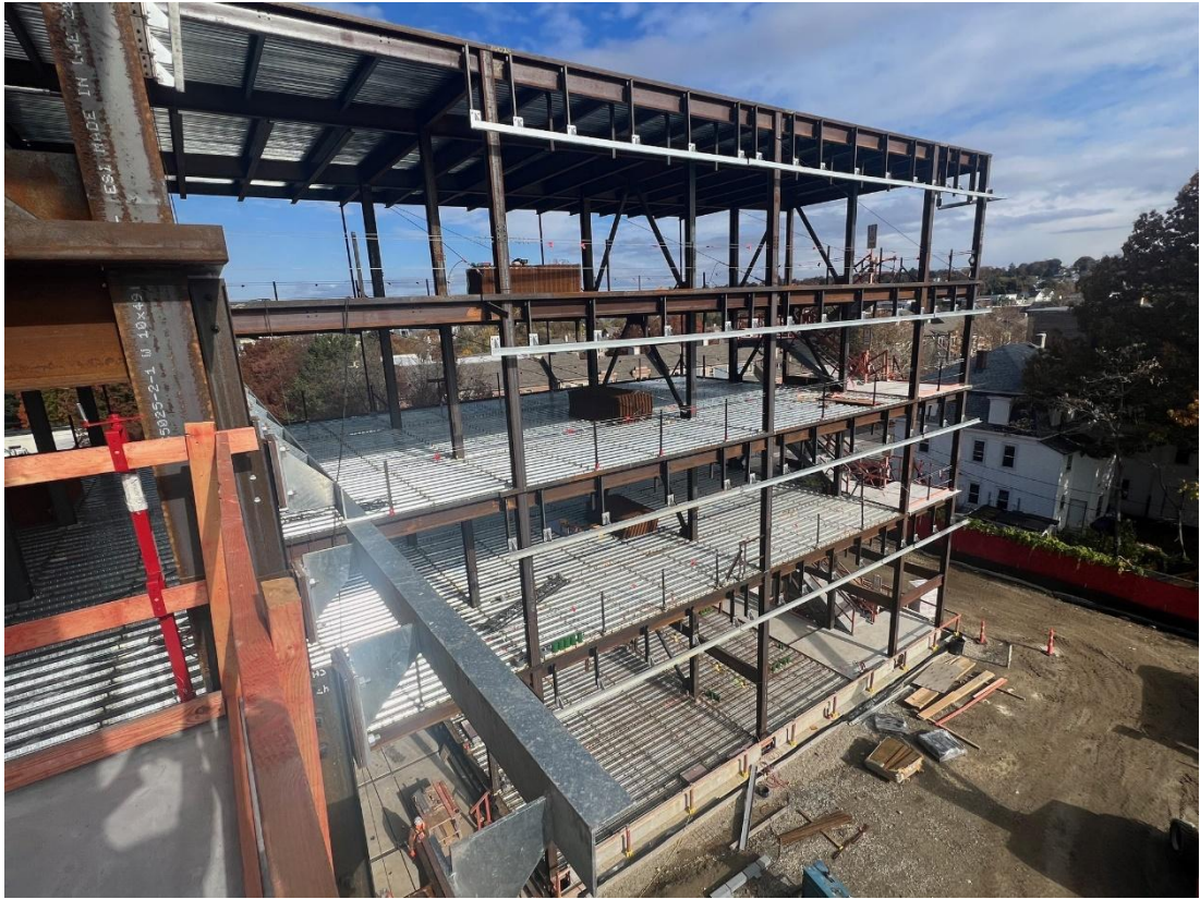
Steel Erection – Level 1 thru Roof
