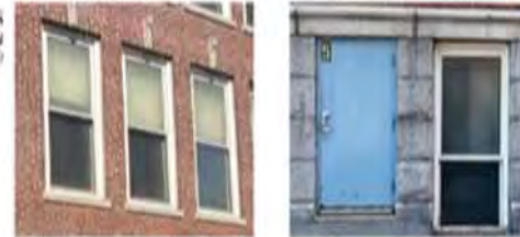
Windows & Doors Remove and replace (typical throughout)
