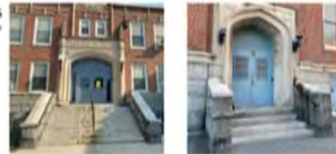
Stairs remove and replace
