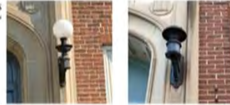
Light Sconces Two per entry, reuse in situ
